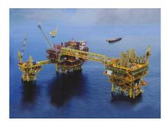
Production Operations utilize fixed offshore platforms and subsea pipelines, with gas processed and exported primarily through pipelines to Thailand. The estimated current production rate of Yetagun is 29.9 MMSCFD.
